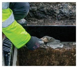
The environmentally friendly alternative to resin-based materials, specifically formulated for the bedding of all access covers.
