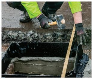
Our HAPAS approved market leading bedding mortar now with added fibres for superior strength gain. Ideal for use with all access covers, as well as for the bonding of granite setts, flags and bedding kerbs.
