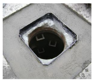
Designed for thick section repairs, haunching reinstatements, ironwork backfilling and commerical sign/post installation.
